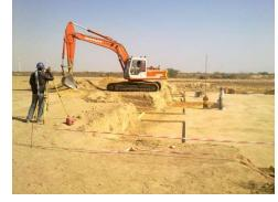
addition to locating improvements, easements, building lines, and encroachments found on the subject property. The corners of the property are physically located, and, if necessary, new corner monuments are installed. Stake surveys are recommended for real estate transactions involving complex commercial and industrial properties, and whenever the survey is to be used for new construction.
